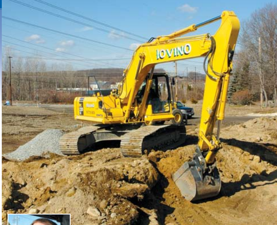
Operator Bob Gettman uses a PC220LC-7 excavator to dig a foundation at a new 10-home development in Burlington, Mass. Iovino crews put in the road, along with sewer, water, drainage, electrical and gas lines. "We were sold from the beginning on Komatsu excavators," said Owner/President Richard Iovino. "It's been our experience that they have more power than competitive brands through the entire digging cycle."
