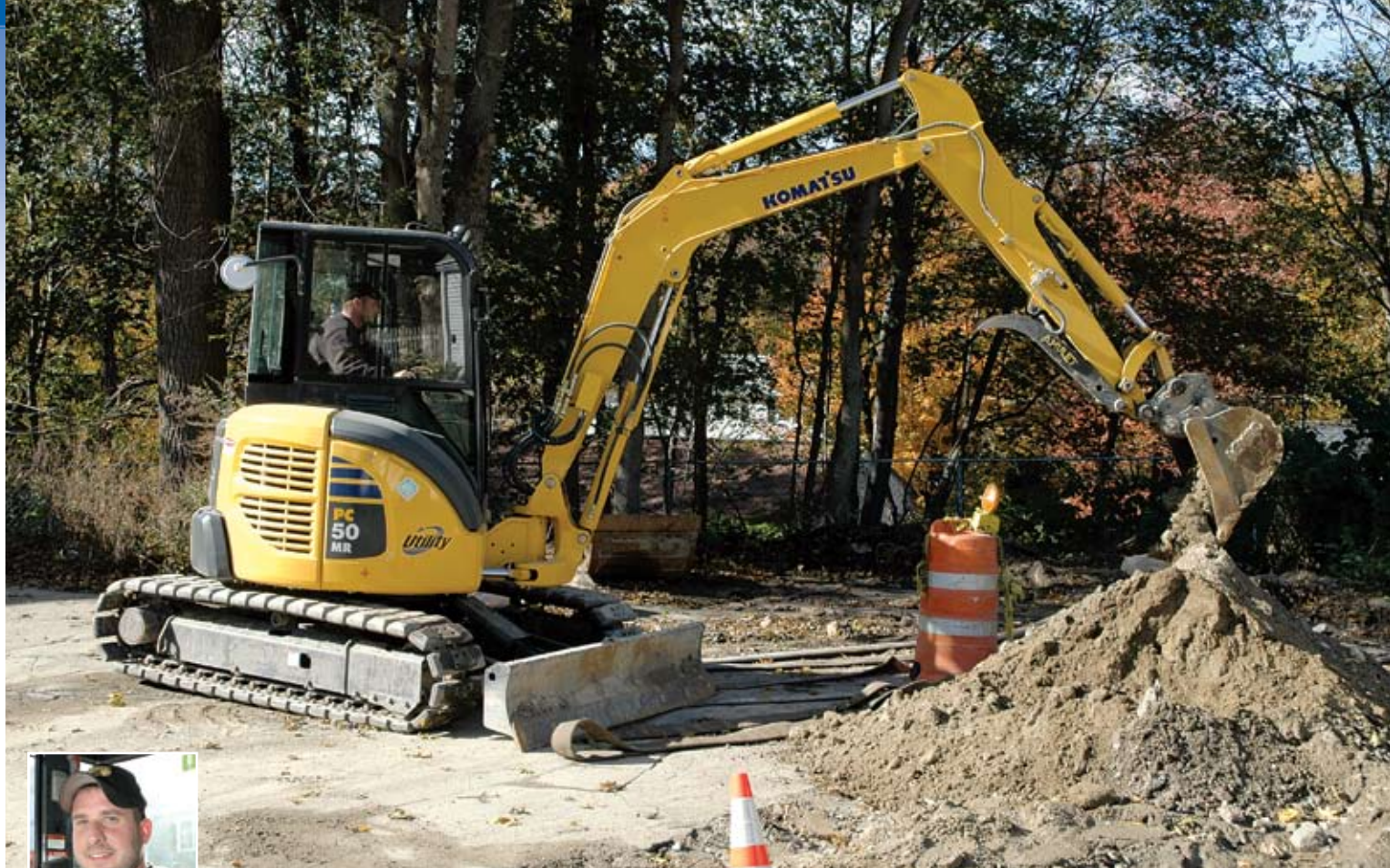
Foreman T.J. Whalen is at the controls of Braintree's new Komatsu PC50MR compact excavator. The town used the PC50 to lay 450 feet of new eight-inch water main line and install service to home owners and a new fire hydrant last fall. "It's awesome for getting in tight spaces," Whalen commented.
