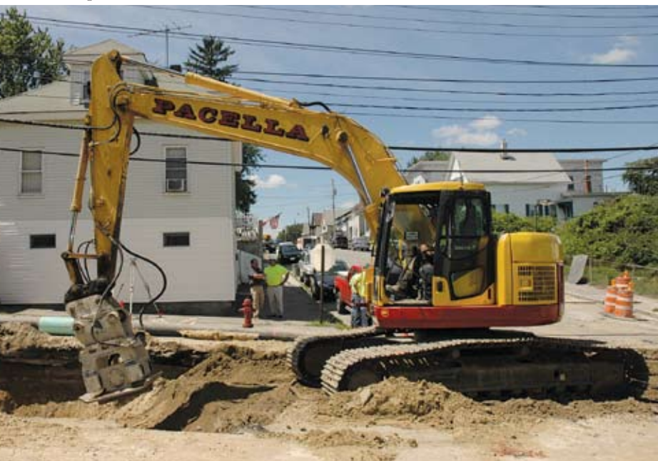
An RJV Construction Corp. operator works a Komatsu PC228USLC-3 excavator with a KHP135 hydraulic compactor attachment.
