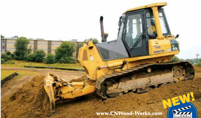
This Albanese Brothers operator uses a Komatsu D41 dozer to stockpile fill material at a job in Manchester, N.H.
