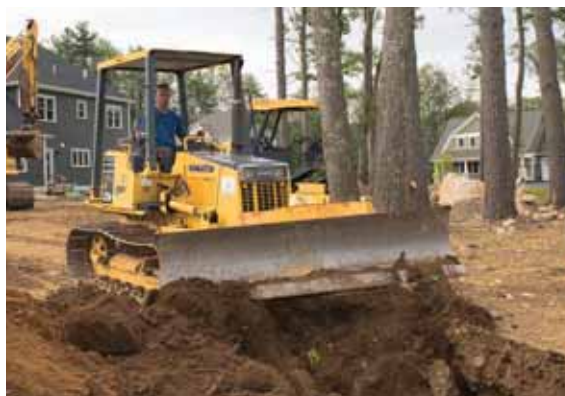
Operator Tim Angelli uses a Komatsu D21P dozer to grade a jobsite.
