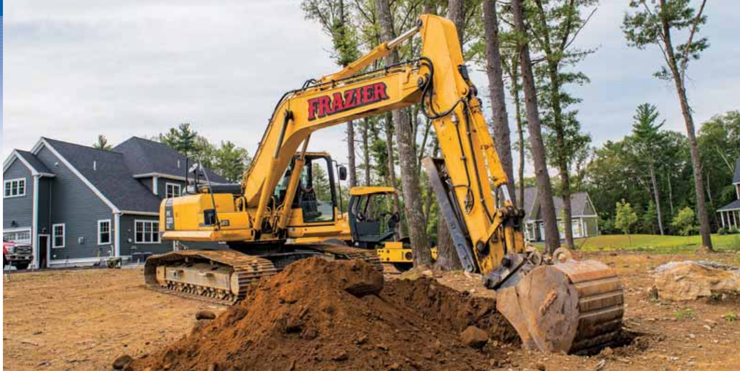
A Frazier Construction operator uses a Komatsu PC220LC excavator to dig a foundation on a residential project in northeast Massachusetts. The company also owns a Bomag BW 177 roller, which it will use later on this job.
